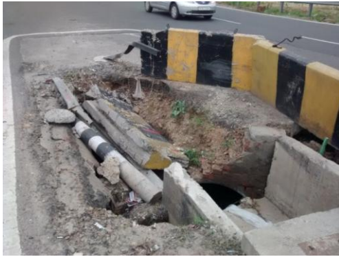
Fig 7: Dangerous Island with open drain
