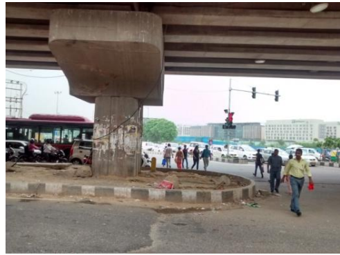
Fig 8: Unpaved Median Nose
